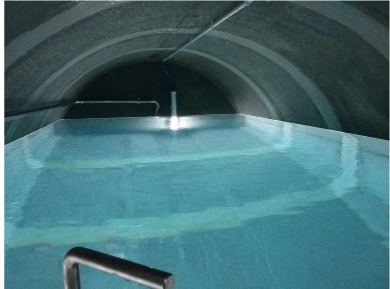
Reservoir in Elementbeton
