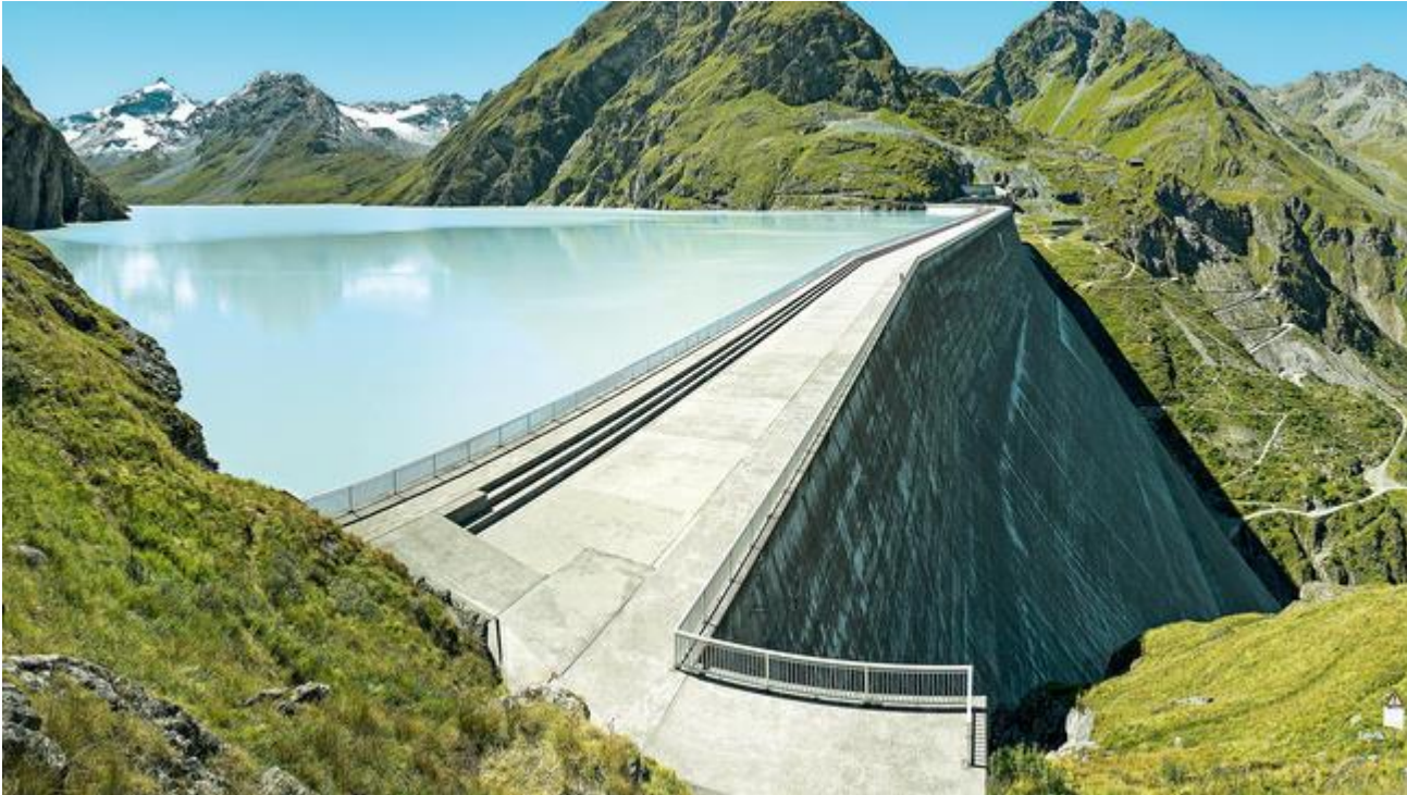
Grand Dixence Staumauer 1953 - 1961
