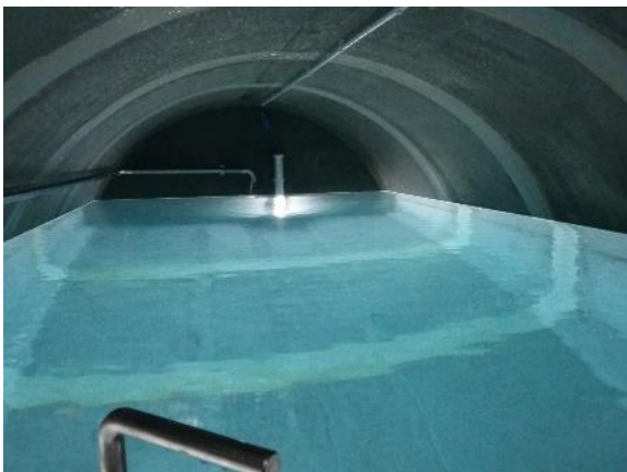
Foto 5: Reservoir in Elementbeton
